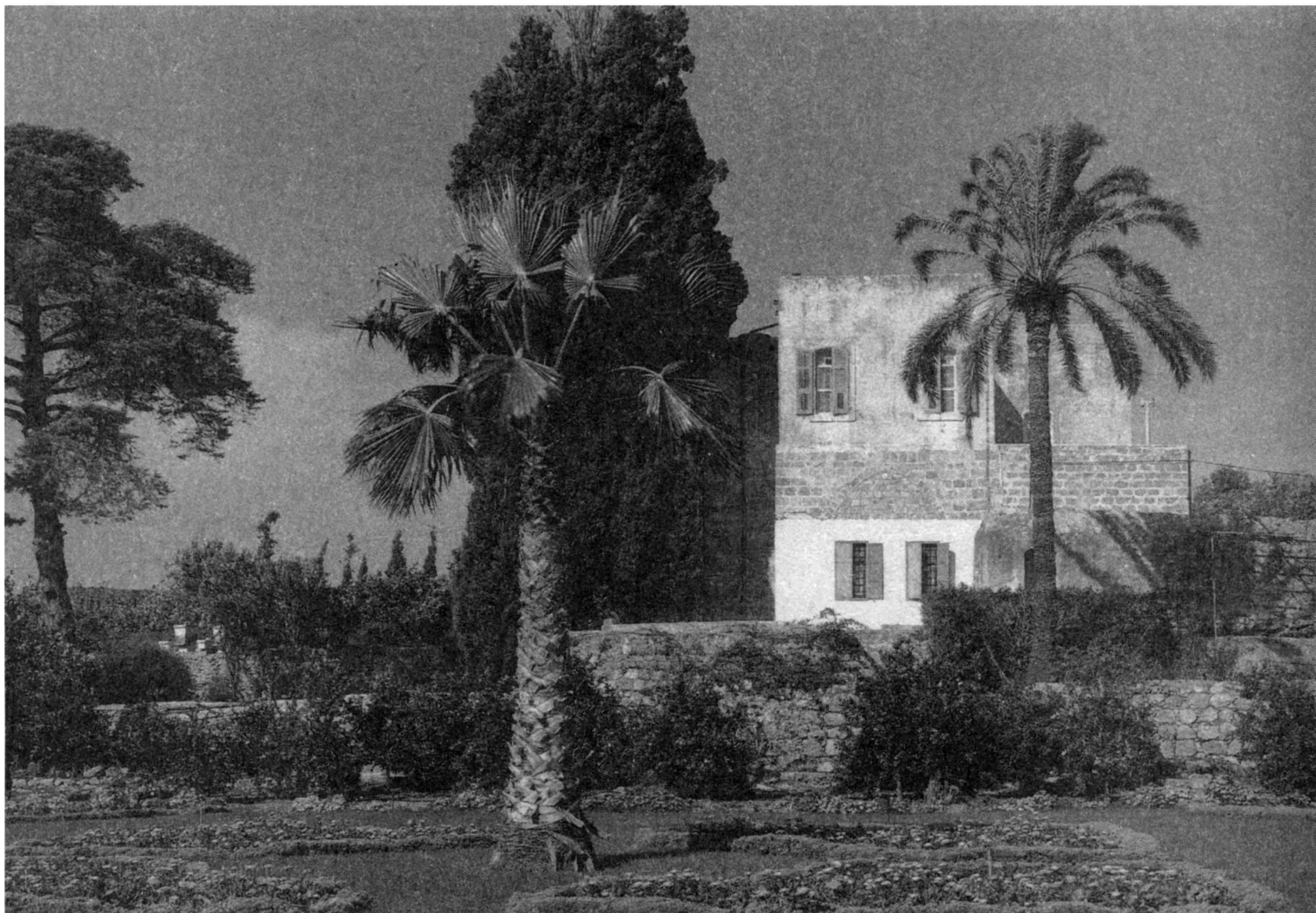
The Mansion of Mazra'ih after restoration
