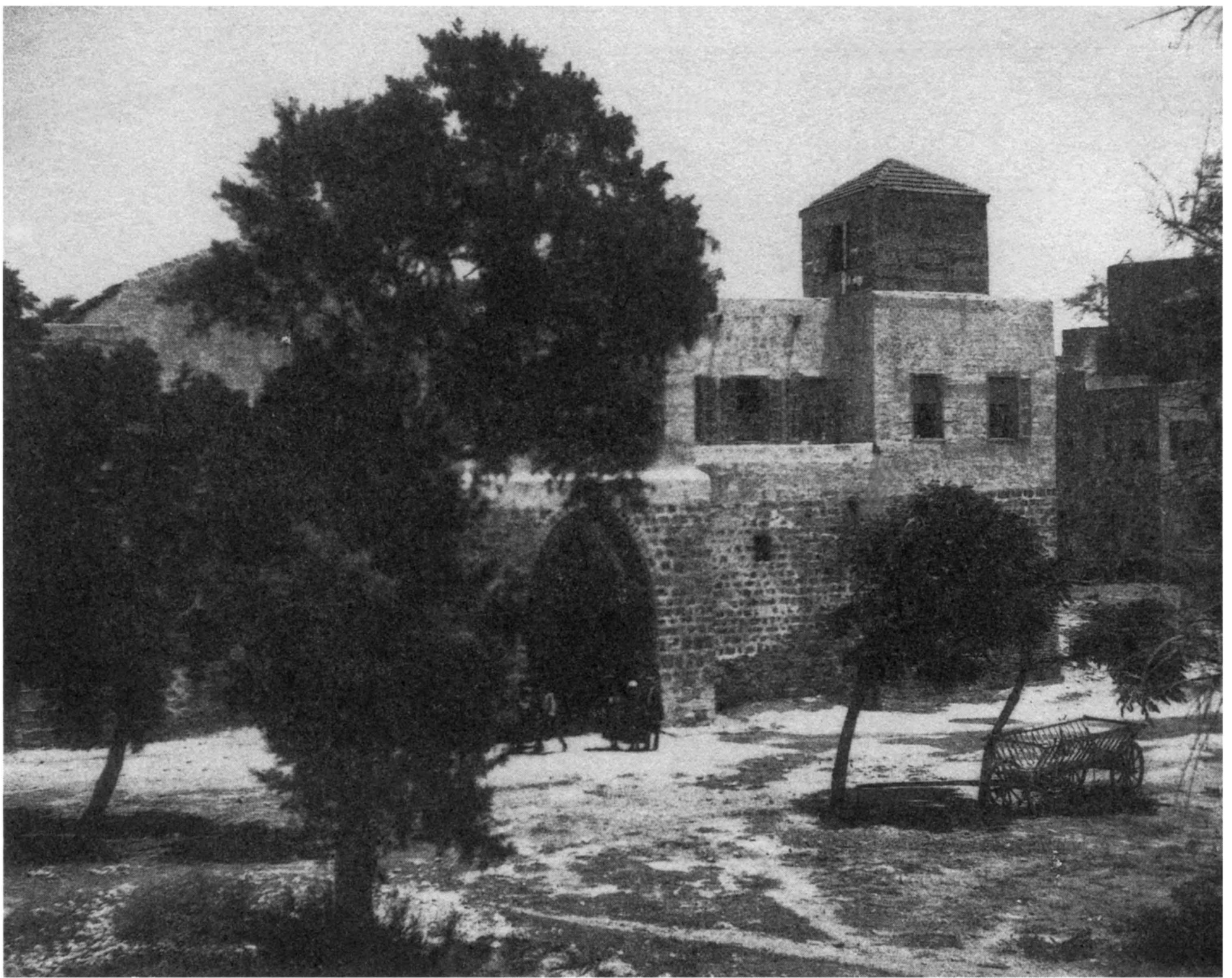
The House of 'Abdu'lláh Páshá The wooden cabin was added by the Master
