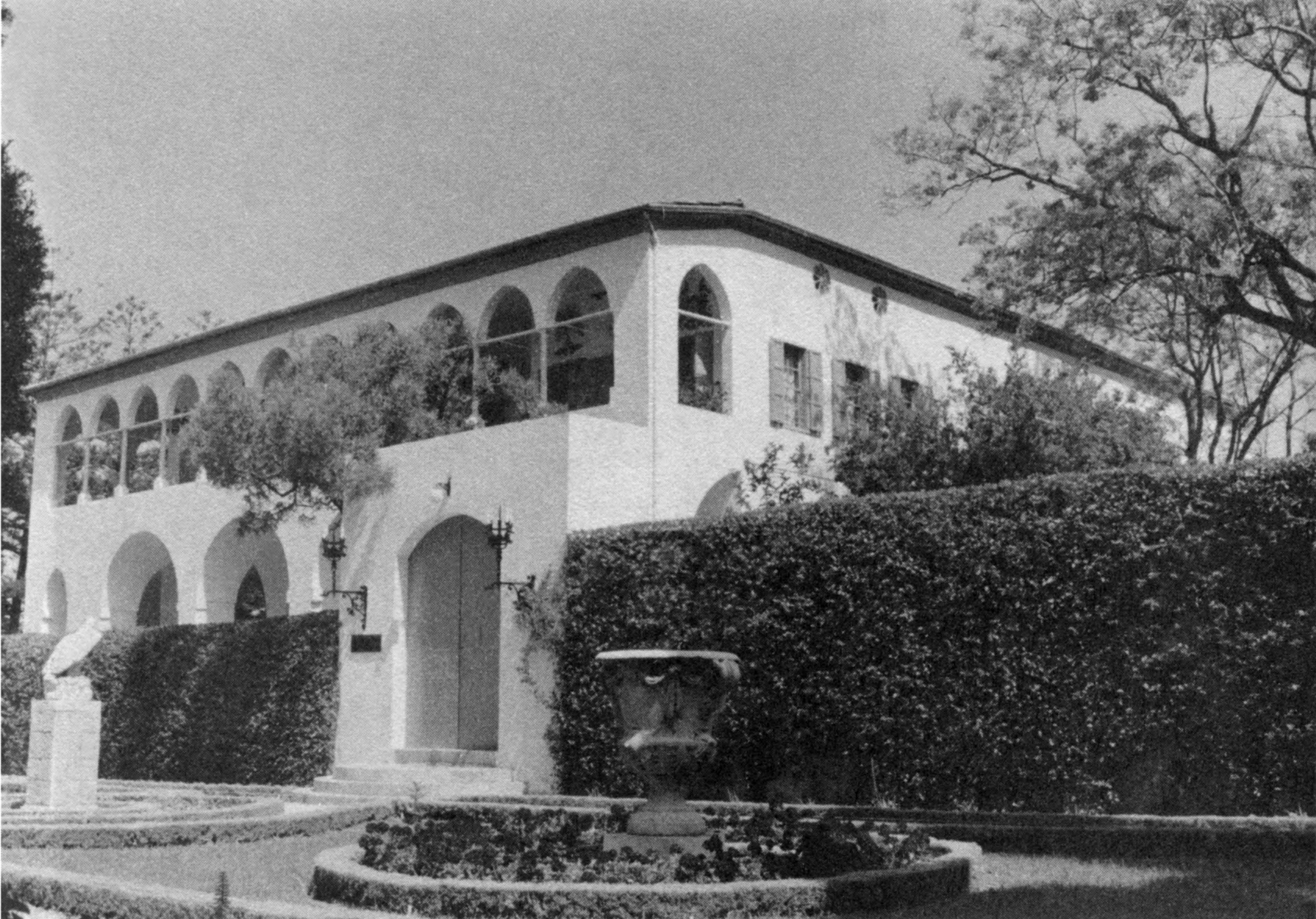
The Mansion of Bahjí restored to its original condition
